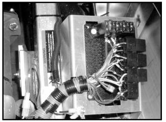
Figure 11c-9 Electrical Component Mounting Plate
