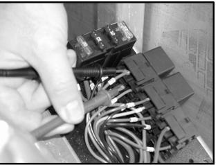
Figure 11b-13 Start Relay Contact Test
