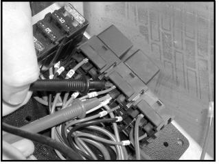
Figure 11b-15 Differential Relay Contact Test
